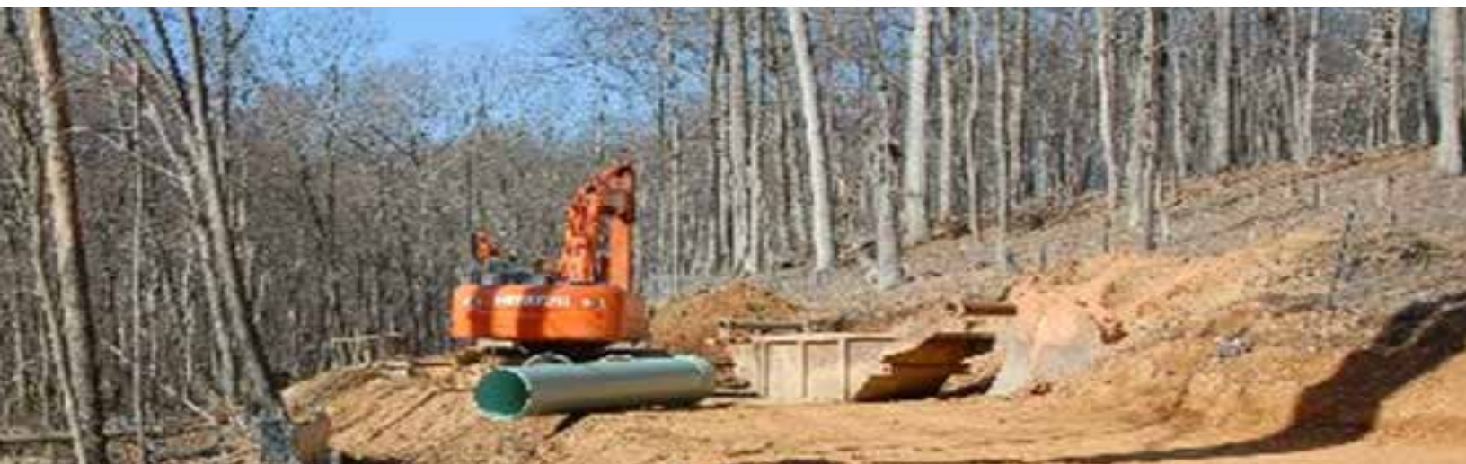
Pipeline installation over protected ground surface
