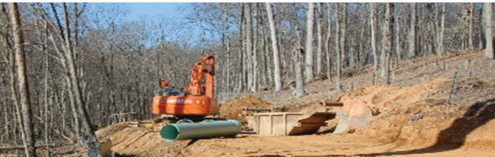
Pipeline installation over protected ground surface
