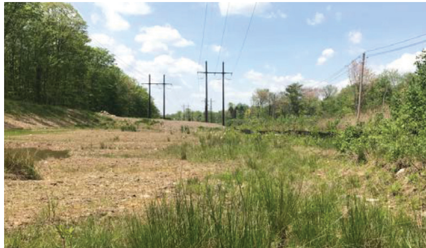
Wetland mitigation under electric transmission line
